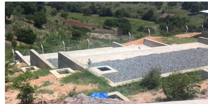
Planted gravel or sand filter (post -WWT part)
